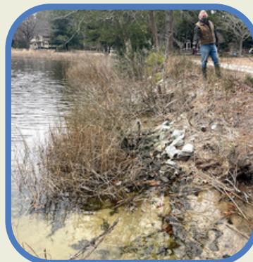
Figure 2: Eroding shoreline at ABTB (2021)
