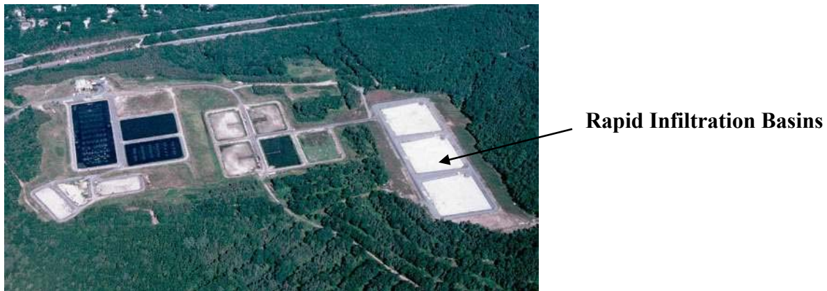
Figure 5-1: Wastewater Treatment Plant with RIBs
