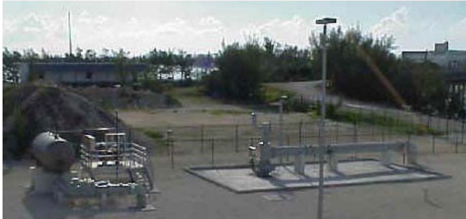
Figure 6-2: Typical Underground Injection Well Head
