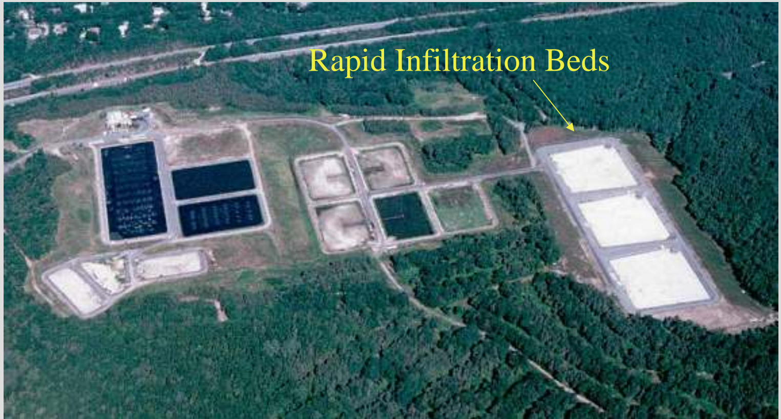
Falmouth, MA – 0.8 mgd facility
