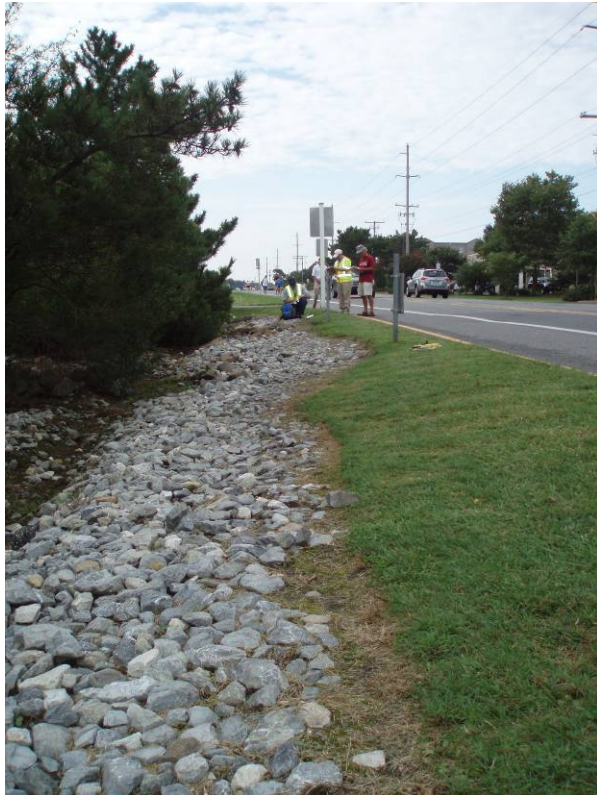
Figures 1&2: Existing Riprap Ditch to be converted into a Forebay
