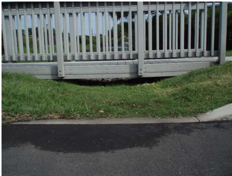
Figure 3: Parking Area discharging to the wet pond
