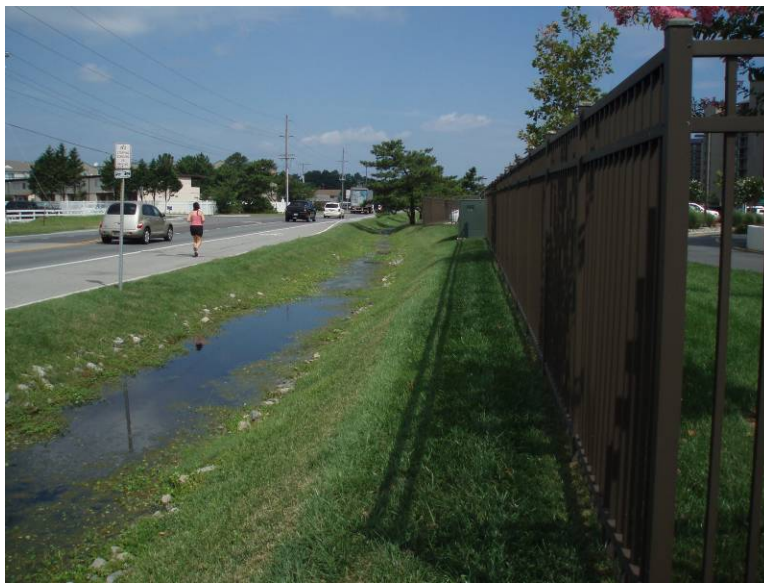
Figure 3&4: Existing Vegetated Ditch (Ditch 3)
