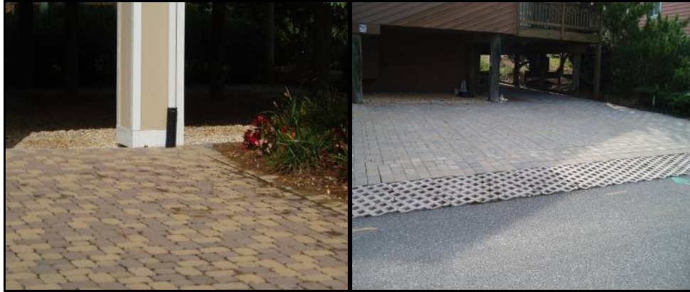
Figure 7. Many impervious surfaces utilized for driveways within the neighborhoods are similar to the design of permeable pavers. Both photos are from N3 (South Bethany). The photo on the right appears to have permeable pavement between the driveway and the right of way, but the base of the pavers is actually impermeable.
