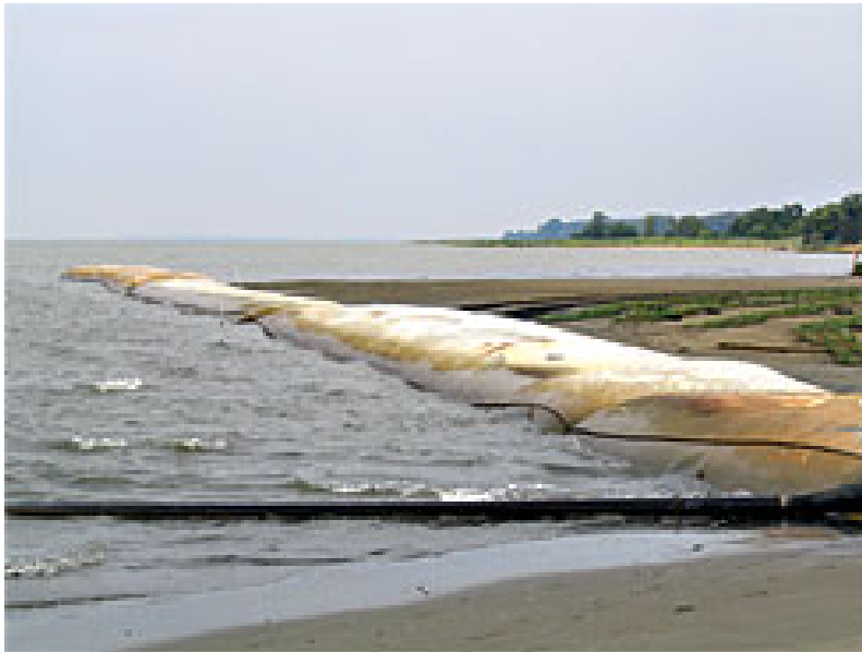
Geotextile Tube Containment
