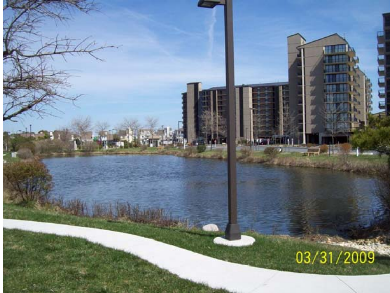
Figure 1&2: Existing wet pond at Sea Colony
