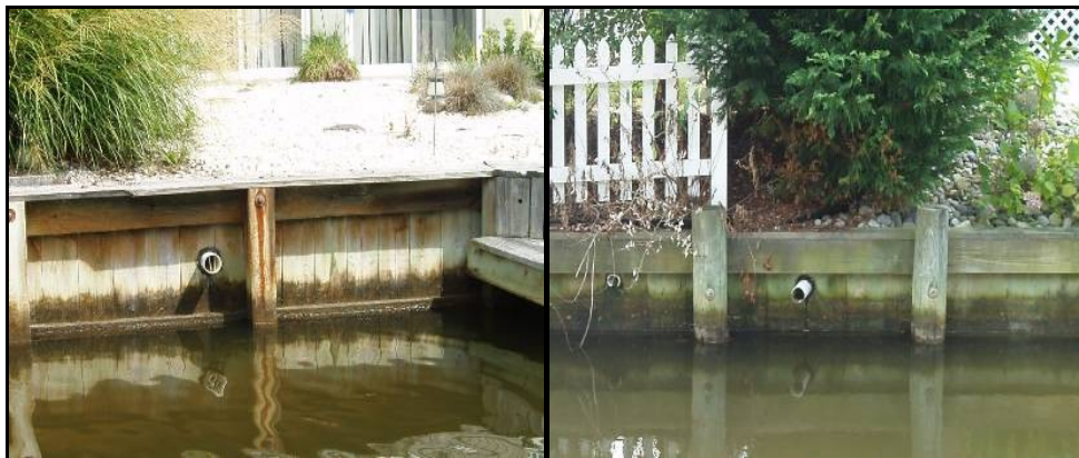
Figure 4. Examples of rooftop downspout and outdoor shower discharge directly into the Anchorage Canal from N4 (South Bethany).
