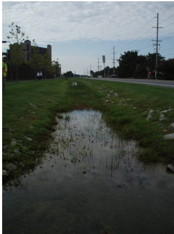
Figure 4: Existing Vegetated Ditch showing the side slopes that are proposed to be converted into filter strip
