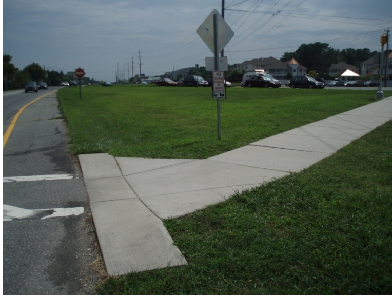
Figure 4: Retrofit Site as viewed from pedestrian cross walk connecting Sea Colony
