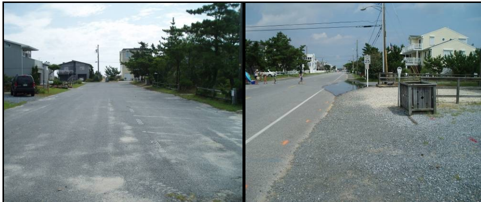
Figure 8. Examples of parking utilized more heavily during the tourist season, where permeable pavers could be installed to help reduce impervious surface within the drainage area. Left – impervious paved parking spaces in N3 (Middlesex Beach) and Right – gravel metered parking spaces along Pennsylvania Ave at N1 (Bethany Beach).
