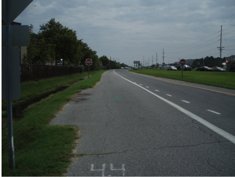
Figure 1&2: Retrofit Site as viewed from Sea Colony Entrance
