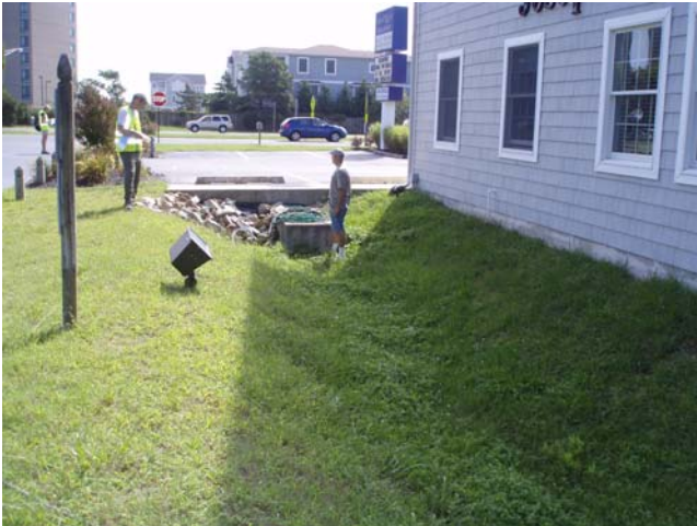
Figure 1: Bioretention area between Short Road and law office.
