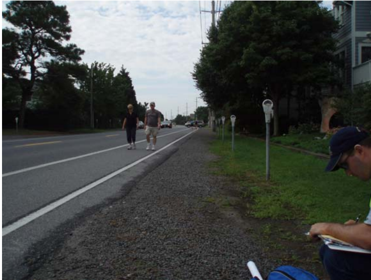
Figures 1&2: Existing Gravel/grass overflow parking to be replaced by reinforced turf overflow parking
