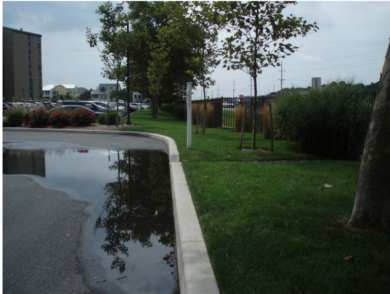
Figure 1&2: Curb Openings at Sea Colony Parking Lot
