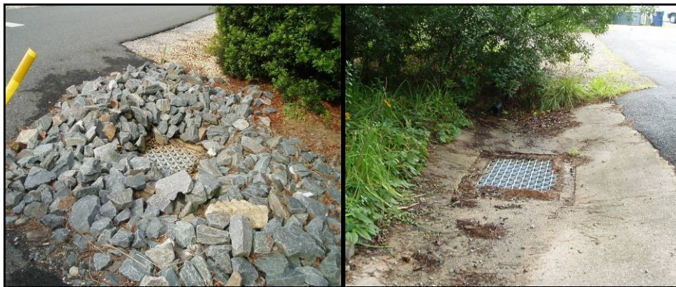
Figure 9. Inlets surrounded by rip-rap and concrete in N4 (South Bethany) that can be modified to remove the impervious cover and include grass/native vegetation pretreatment.
