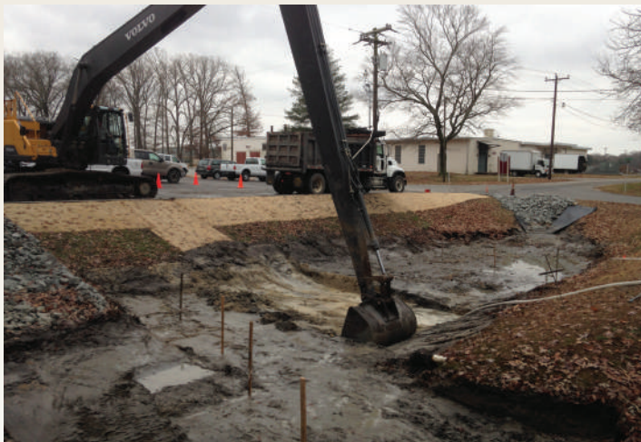
Construction was completed on the new bioretention area in December 2016
