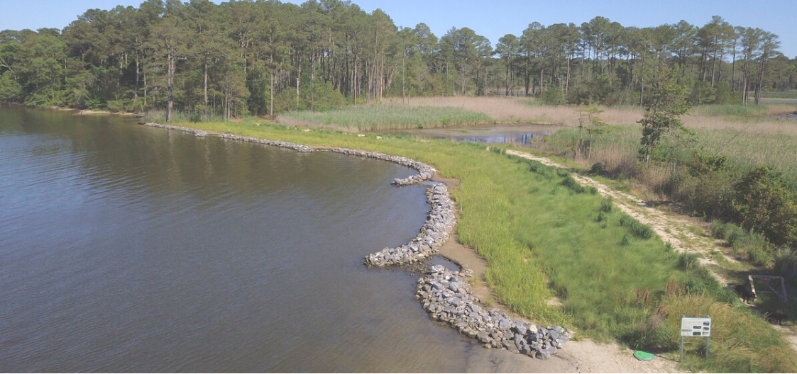
A living shoreline was installed at Sassafras Landing to reduce erosion and restore habitat.
