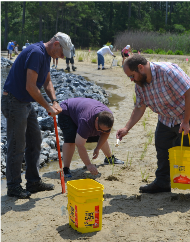
Volunteers helped install more than 5,000 plants at the SassafRAS Landing living shoreline site.
