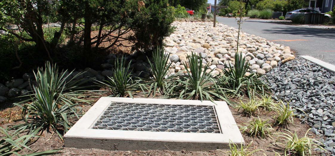
A rain garden and infiltration trench installed in the Sandpiper Pines neighborhood.
