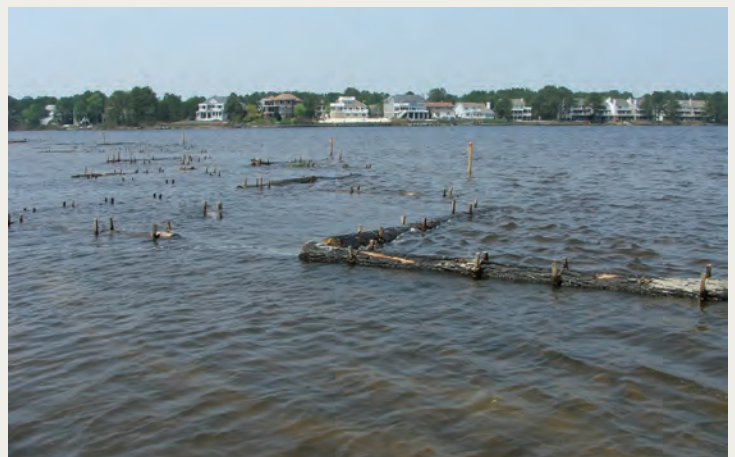
This photo shows the quieter water on the marsh side of the log breakwater structure.
