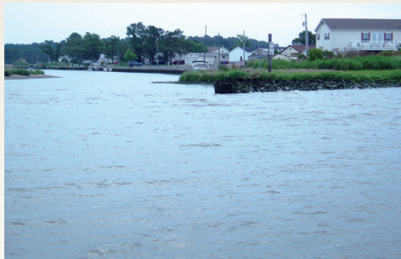
View of marina entrance after removal of the derelict bulkhead and pilings.
