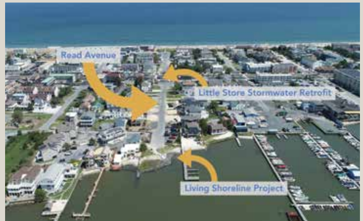
Dewey Beach and its Read Avenue, marked and labeled with project sites, are bordered on one side by Rehoboth Bay and the other by the Atlantic Ocean. Photo by Larry Trout, RK&K.
