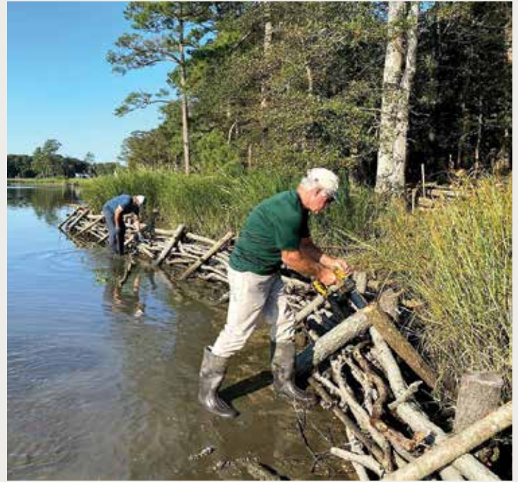
Center Program Manager, Bob Collins, (left) and volunteer, Jerry Daugherty, work on the anchored branch toe.
