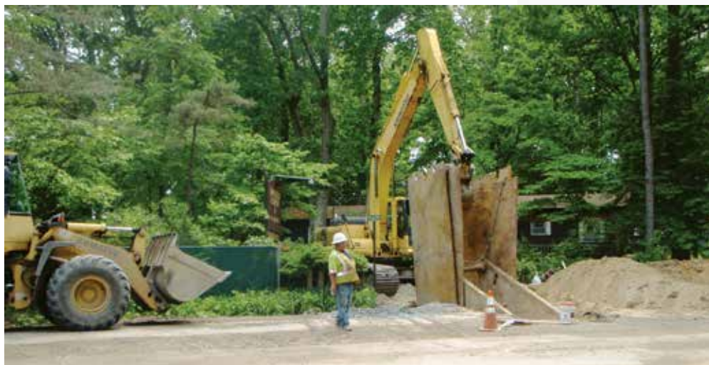
Central sewer expansion on Angola Neck.
