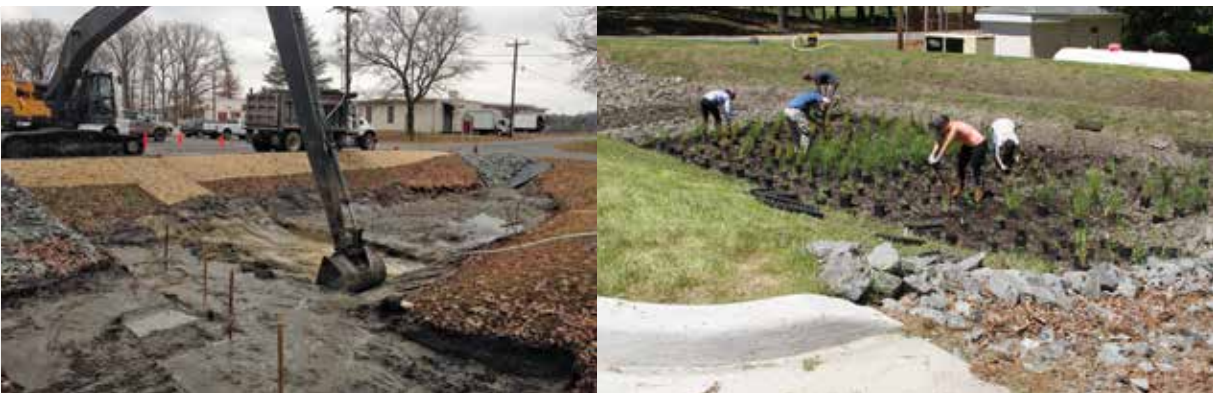
Construction began in late 2016 and wrapped in 2017 with a planting day.
