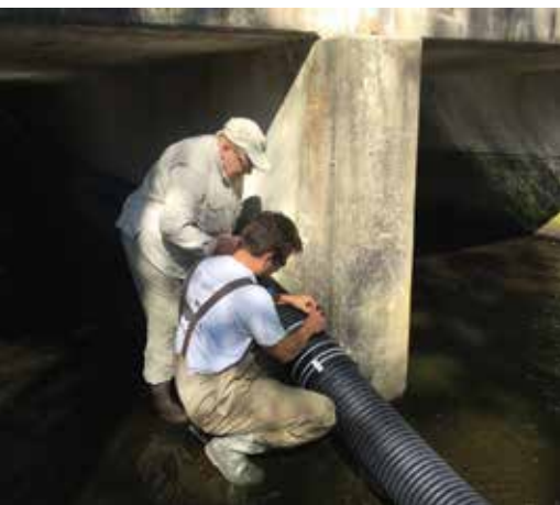
Center Board Chair, Susie Ball, and Environmental Scientist, Andrew McGowan, affix the eelway to a piling of the dam.
