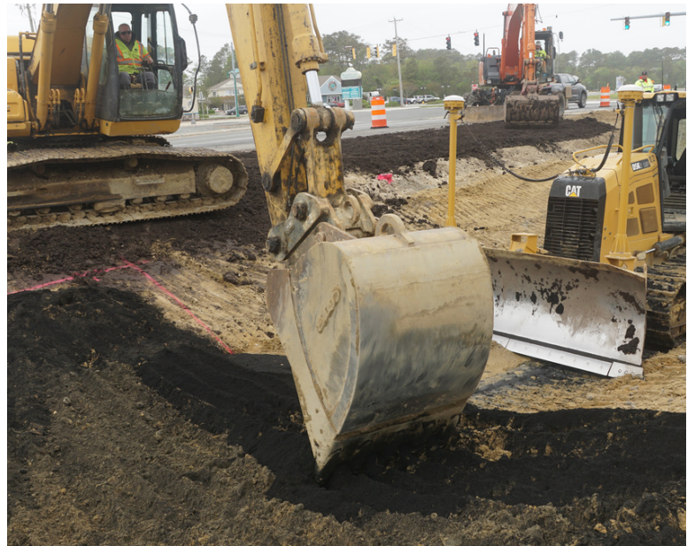
Biochar, the darker material shown in the photo above, was incorporated into the pond and wetland soil.
