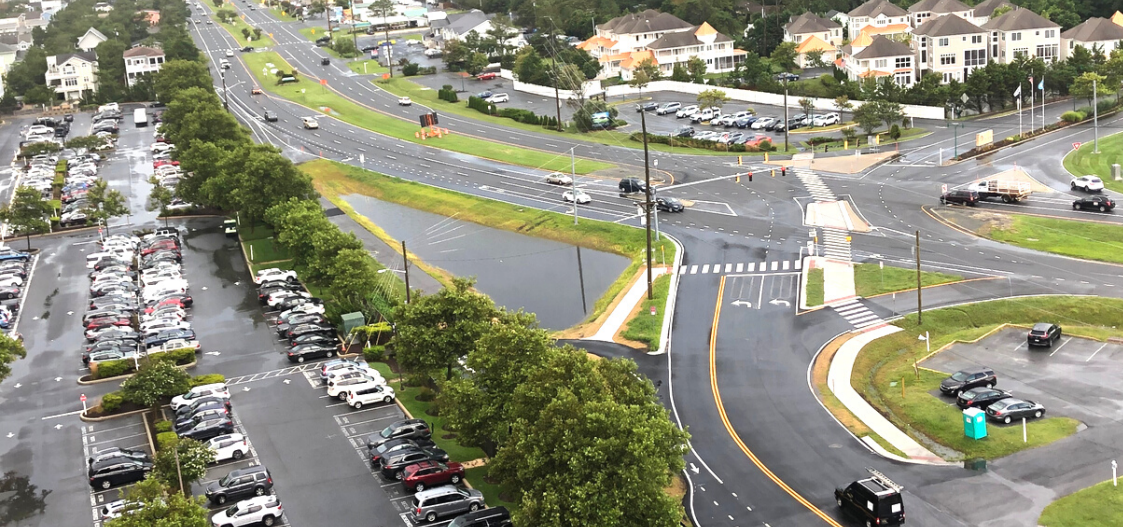
The Anchorage Canal pond immediately after construction.
