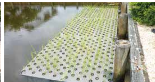
A new wetland installed along a dead end bulkhead
