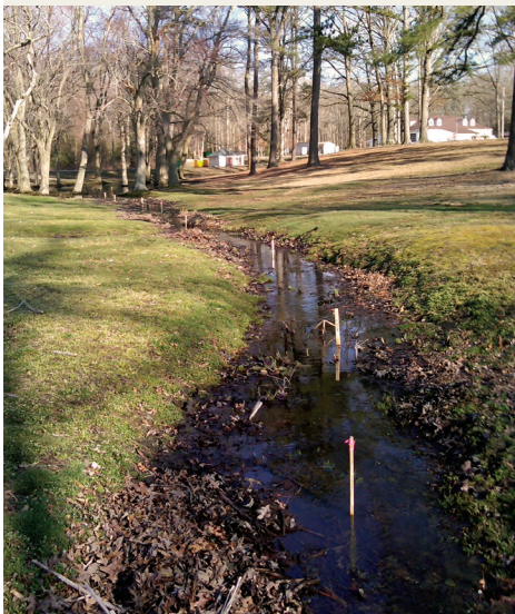
Prior to construction, stakes were placed to identify the centerline of the stream channel.
